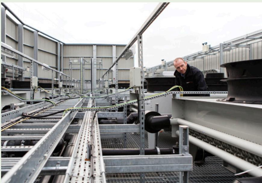
At KDC DUB 1 and KDC DUB 2, closed-circuit cooling systems were implemented which offer peak-efficiency long-term operation. Through this system, there is reduced water loss through evaporation, therefore lowering water consumption and improving energy efficiency.
