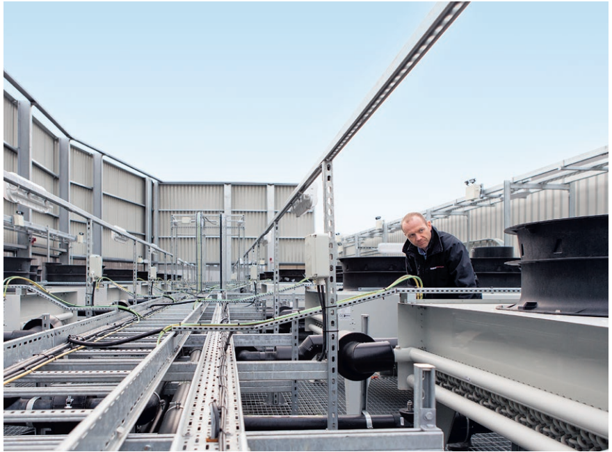
In 2025, Keppel DC REIT was named joint winner of the Energy Impact Award at the DCD Awards in Ireland, recognising its commitment to advancing energy efficiency and sustainability in data centre operations.
