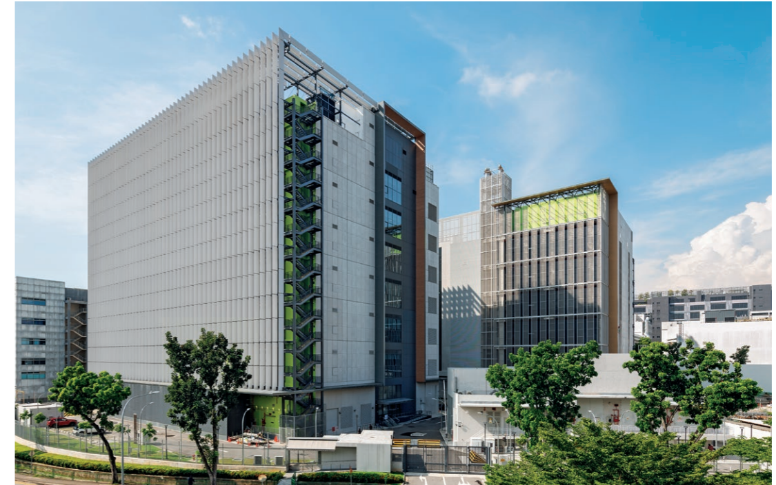
In 2025, Keppel DC REIT acquired the remaining interests in Keppel DC Singapore 7 and 8, achieving full ownership and secured a 10-year land tenure lease extension.
