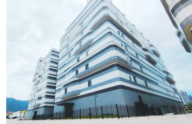
Guangdong Data Centres 2 & 3, China
