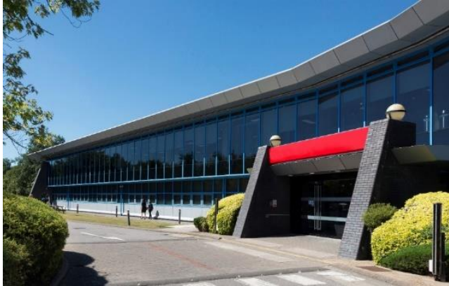
London Data Centre, United Kingdom
