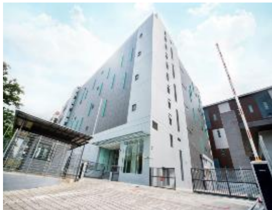
Keppel DC Singapore 5
