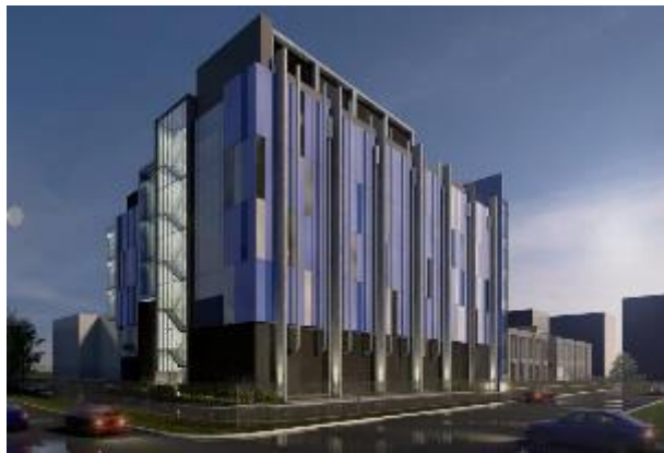
Intellicentre 3 East Data Centre
