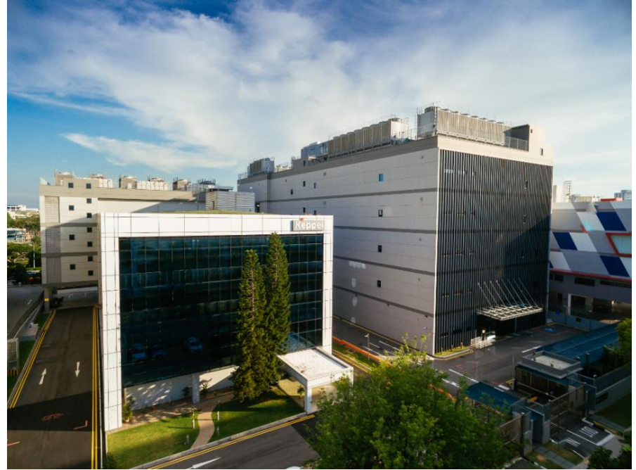
Keppel DC REIT is well-positioned capture value from the data centre industry with its quality portfolio of assets
