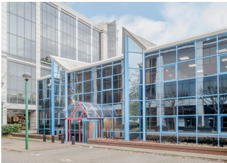
The REIT has colocation data centres as well as master-leased facilities, such as the GV7 Data Centre (in picture)
