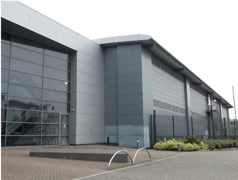
Data centre in Cardiff, United Kingdom
