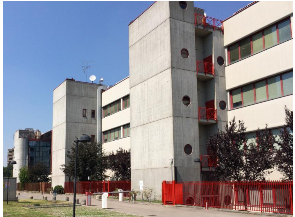
Data centre in Milan, Italy
