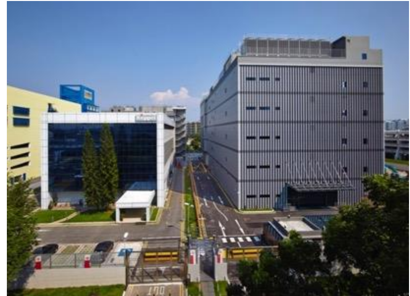
The Sponsor operates five data centre facilities: S25, T25 and T27 (above) in Singapore, Citadel 100 Data Centre in Dublin, as well as Gore Hill Data Centre in Sydney
