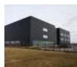
Almere Data Centre 2 (1) Netherlands
