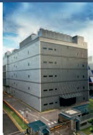
Keppel DC Singapore 3
