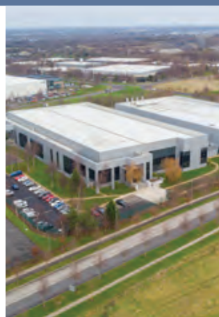
Keppel DC Dublin 1
