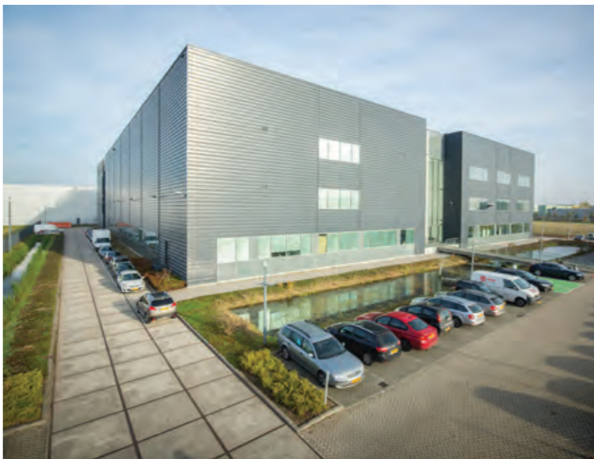
Keppel, together with its private funds, has more than $2 billion worth of data centre assets under development and management that Keppel DC REIT can potentially acquire.
