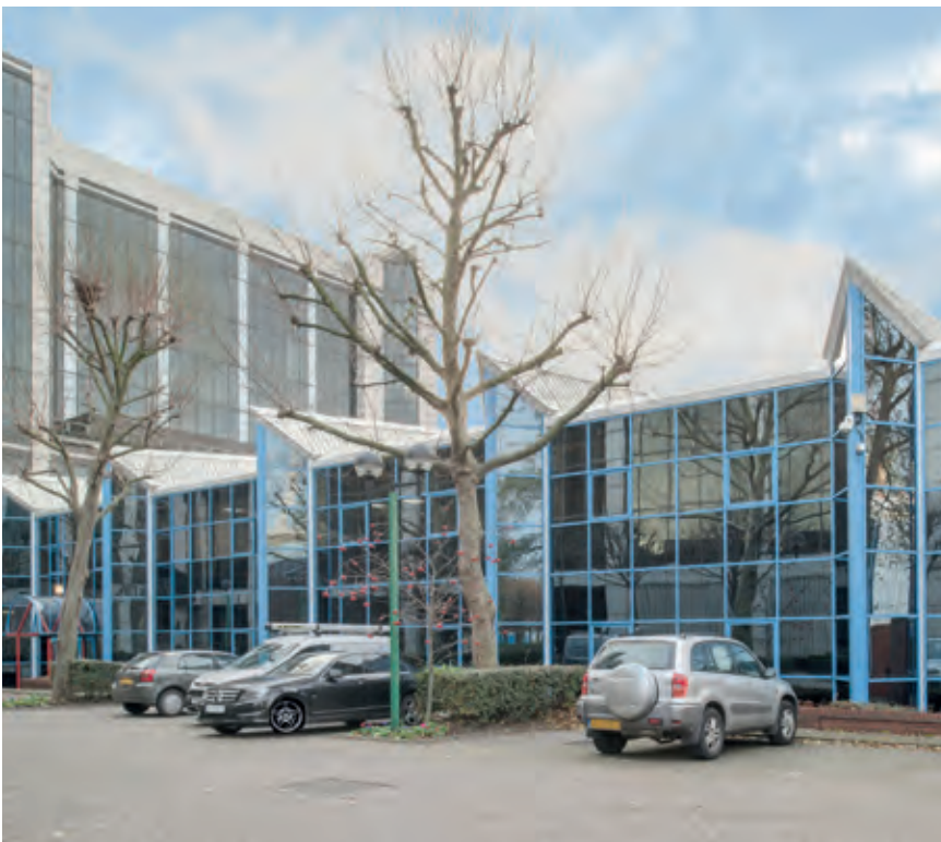
GV7 DC is located in Greenwich View Place, a data centre hub with many operators offering high connectivity services.
