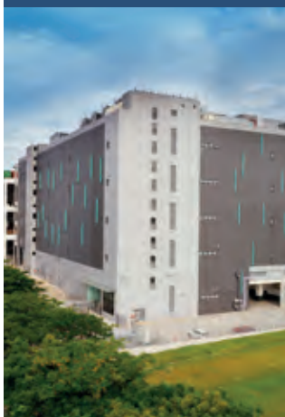
Keppel DC Singapore 5
