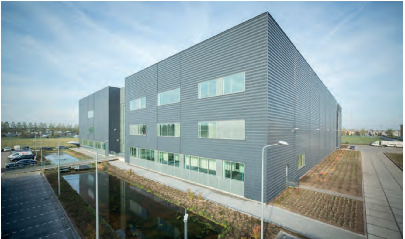
Almere DC is located in the Sallandsekant business park, in the city of Almere, the Netherlands.
