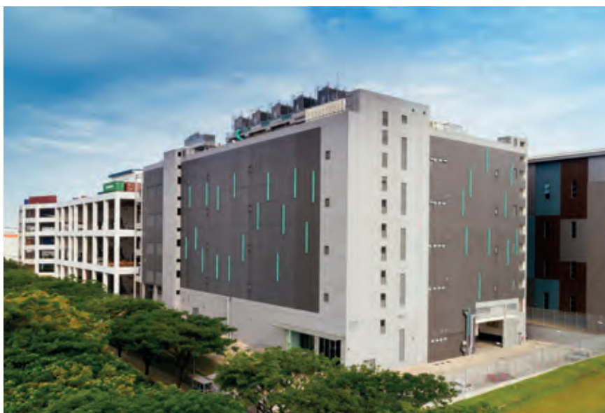
Keppel DC Singapore 5 is located in Jurong, one of the largest clusters of data centres in Singapore.
