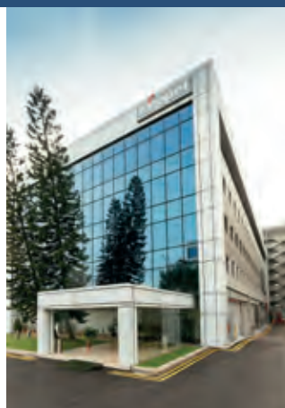
Keppel DC Singapore 2
