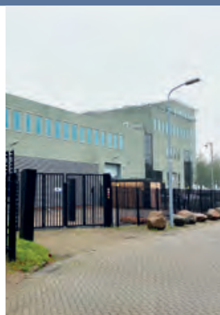
Amsterdam Data Centre
