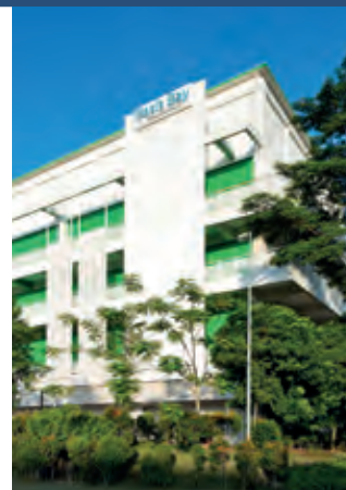
Basis Bay Data Centre
