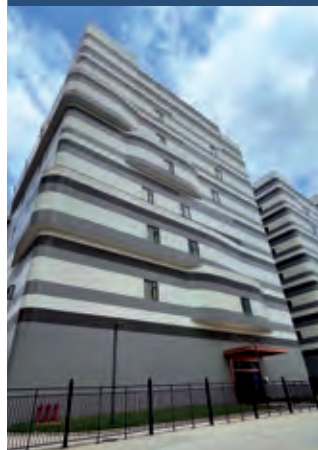
Guangdong Data Centre 1
