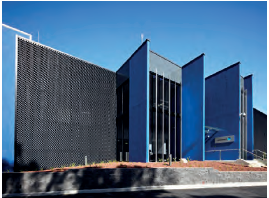
Intellicentre Campus is located within Macquarie Park in the north of Sydney, and is 12km away from the central business district.
