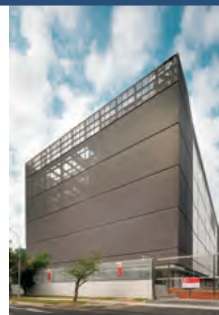
Keppel DC Singapore 4
