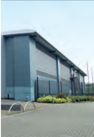
Cardiff Data Centre
