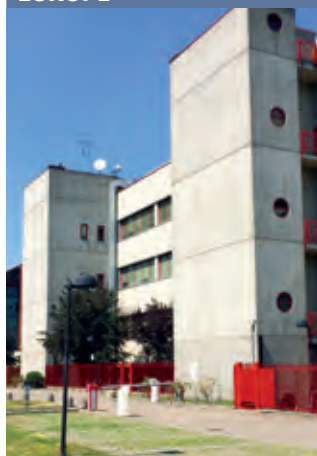
Milan Data Centre
