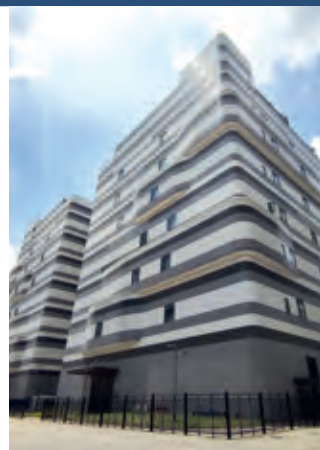
Guangdong Data Centre 2
