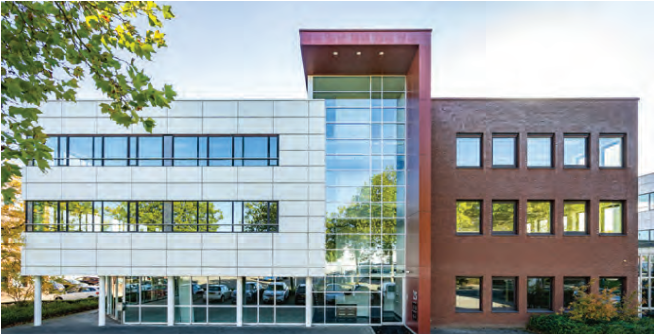
Eindhoven DC comprises two shell and core data centre buildings as well as a warehouse and an ancillary office building in De Hurk, the largest business park in Eindhoven, the Netherlands.
