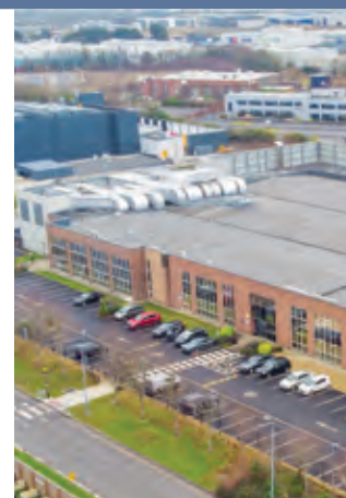
Keppel DC Dublin 2
