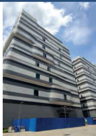
Guangdong Data Centre 3
