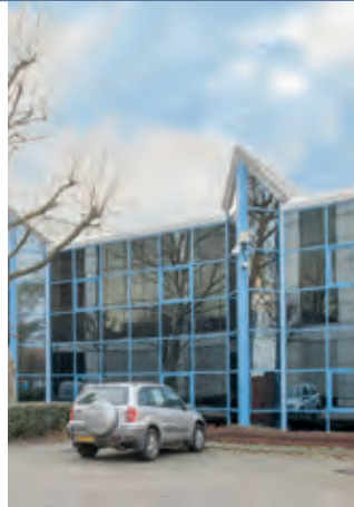
GV7 Data Centre
