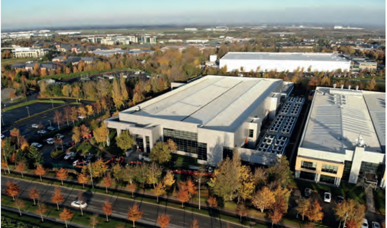
Keppel DC Dublin 2 is an energy-efficient colocation data centre located in the Citywest Business Campus, a prime suburban industrial and commercial location.
