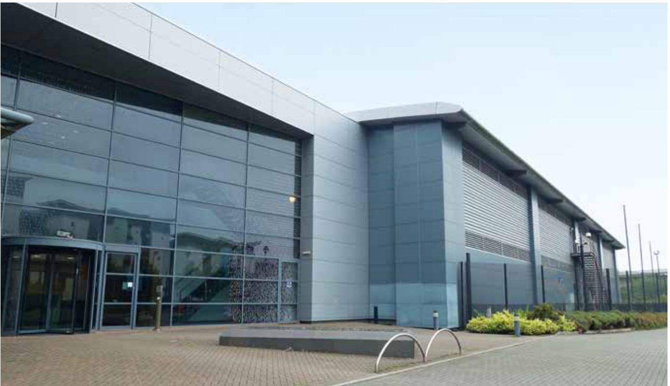
Cardiff Data Centre is strategically situated within the Celtic Gateway Business Park.
