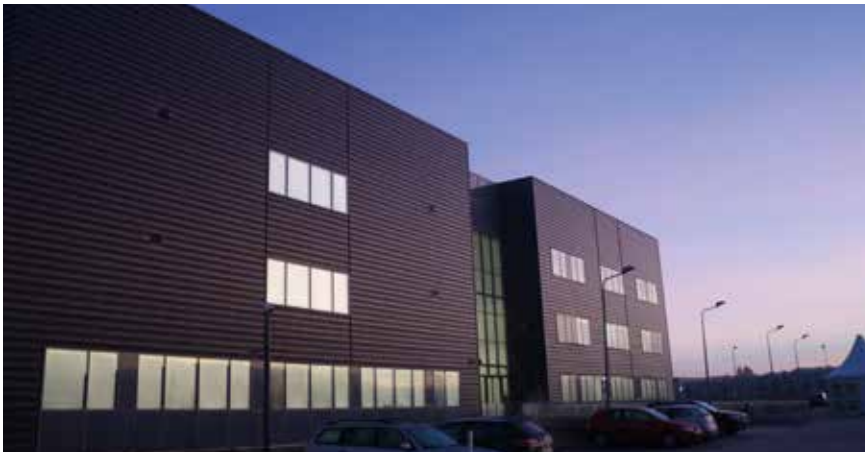
With connection to North America and Europe via submarine cables, Almere Data Centre provides a highly-connected and secure environment for clients.
