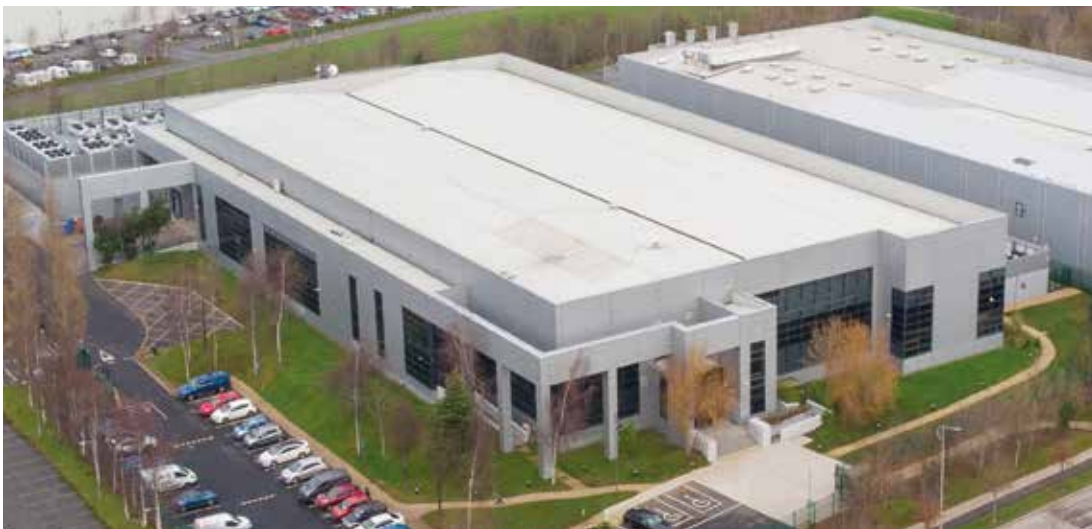
Keppel DC Dublin 1 is located in the Citywest Business Campus, a prime suburban industrial and commercial location in Dublin.
