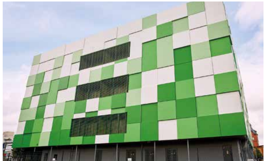
maincubes DC is located within a data centre hub and offers high interconnectivity to the world's leading internet exchange point, DE-CIX.
