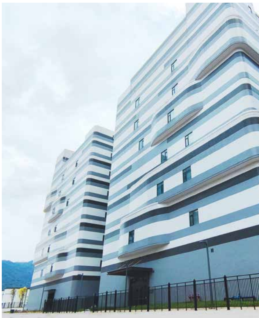
Keppel DC REIT has three data centres in Guangdong, which are designed in accordance with the Code for Design of Data Centre Grade A GB, where Grade A is the highest standard for data centres in China.
