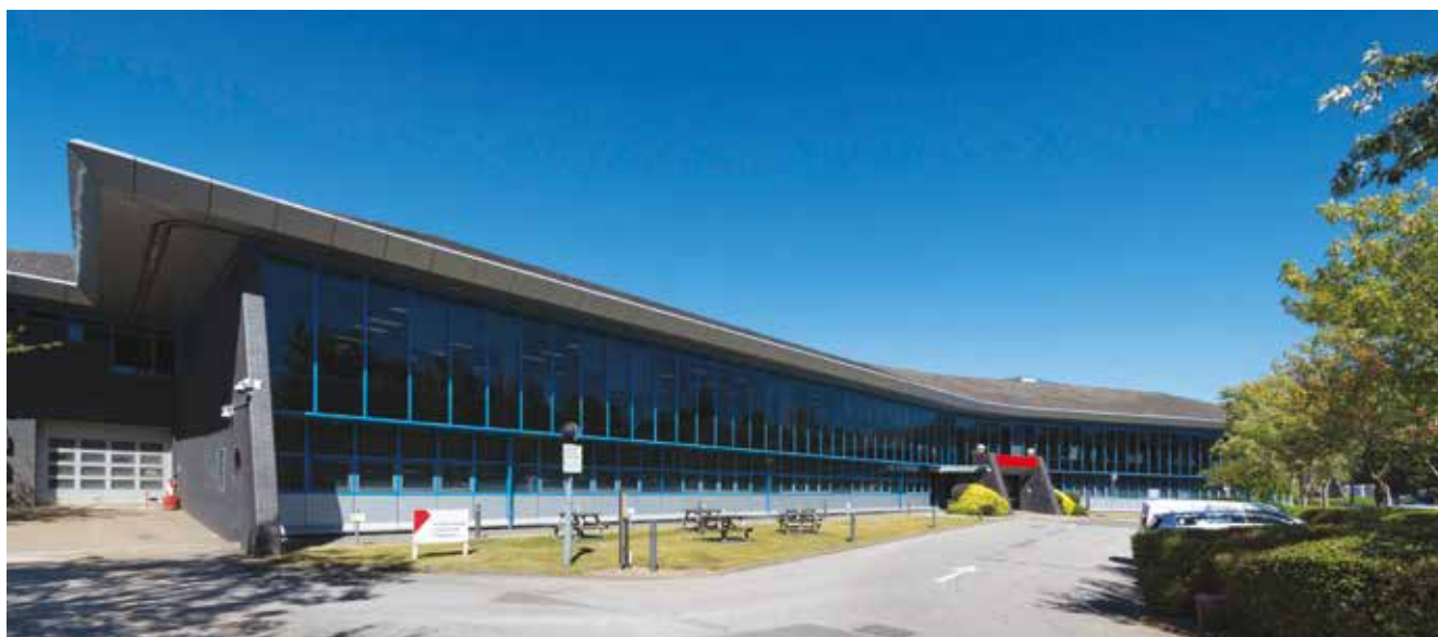
London Data Centre is strategically located in Bracknell, a commercial centre in the Thames Valley, a region considered to be the Silicon Valley of the UK.
