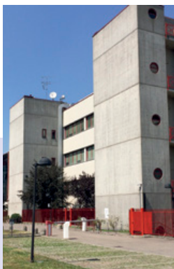
Milan Data Centre
