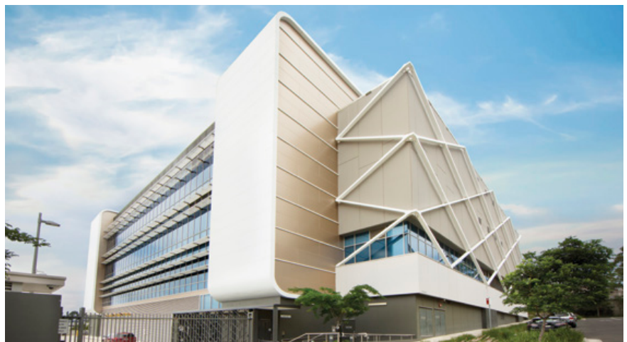
Gore Hill Data Centre is located within the Gore Hill Technology Park in Sydney, Australia.
