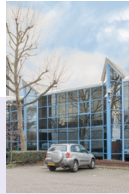
GV7 Data Centre
