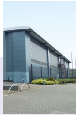
Cardiff Data Centre
