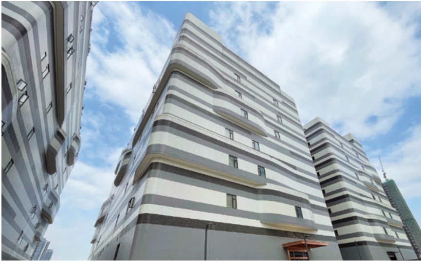
Guangdong Data Centre is located in the Bluesea Intelligence Valley Mega Data Centre Campus in Jiangmen, Guangdong Province in China.
