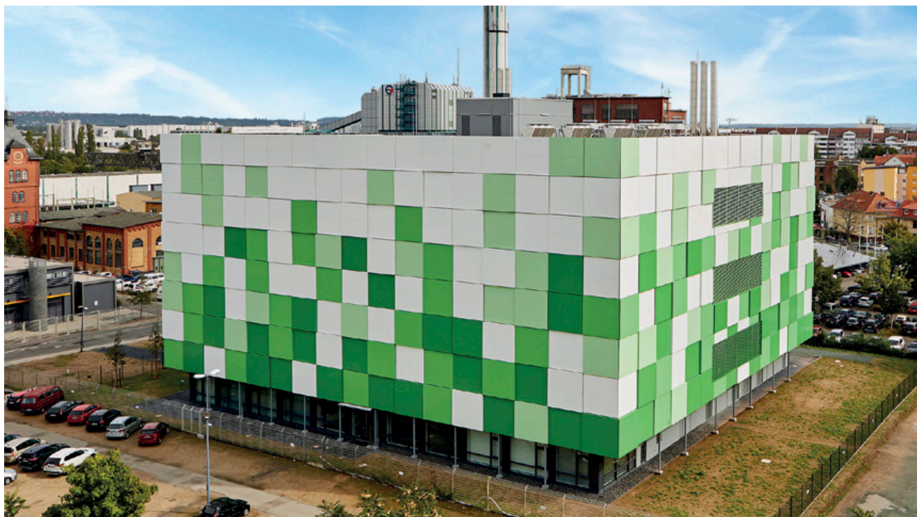
maincubes Data Centre is strategically located within the data centre hub across Frankfurt and Offenbach in Germany.
