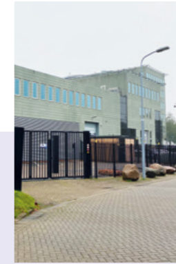
Amsterdam Data Centre
