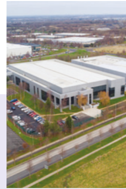
Keppel DC Dublin 1
