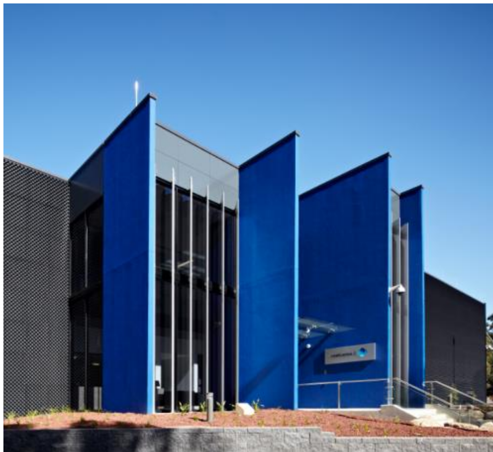
Intellicentre 2 in Australia
